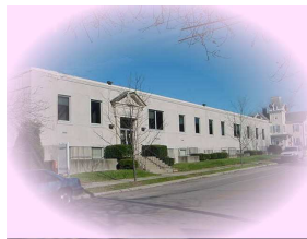
(front view of building from Silver Street)
